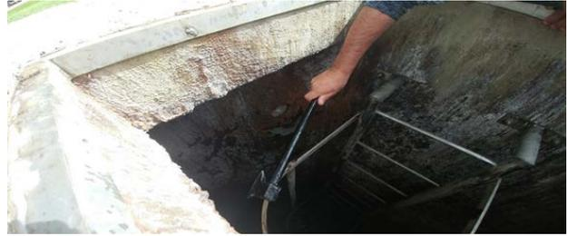
**Fig. 9:** Picture taken in Israel where a system similar to Scenario-2 has shown premature failure after just 5 years in service.
