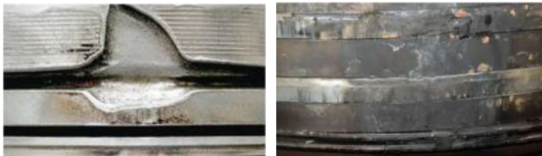
Fig: 1. some of the eroded material due to wear
