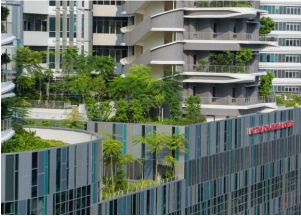
Fig. 16. Implementation of green roofs.
