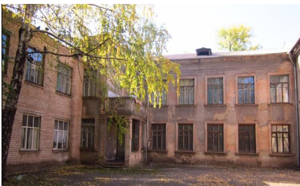
Fig. 4. Hospital building №3, Kryvyi Rih.
