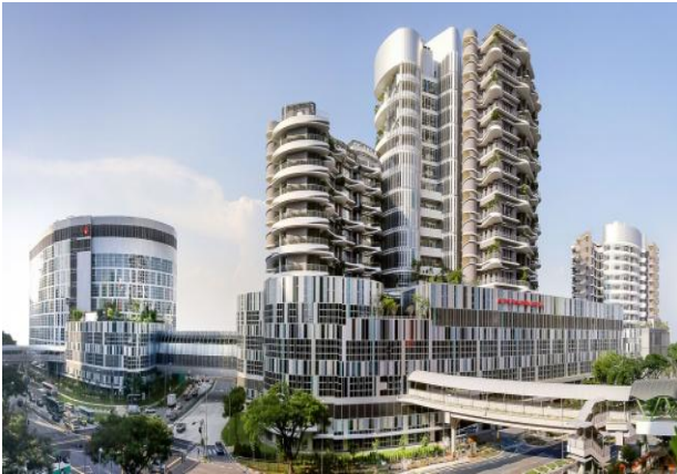
Fig. 6. General view of the hospital complex Ng Teng Fong (NTFGH) & Jurong (JCH).
