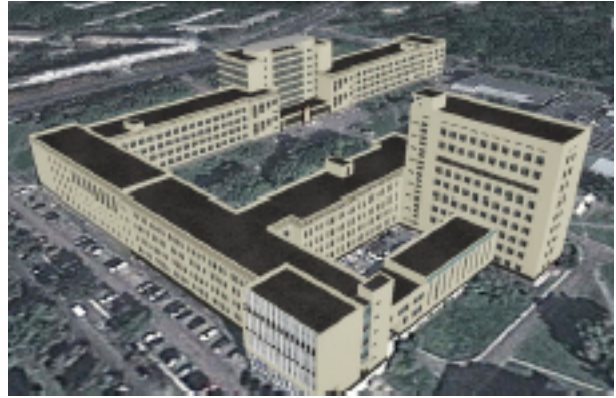
Fig. 5. 3D model of main buildings of the Kyiv National University of Construction and Architecture, Kyiv, Ukraine.
