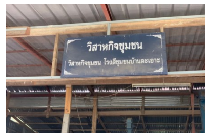
Figure 1. Community rice milling plant.
