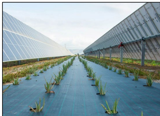
Fig. 13: Inclusion of nursery vegetation between rows of modules.
