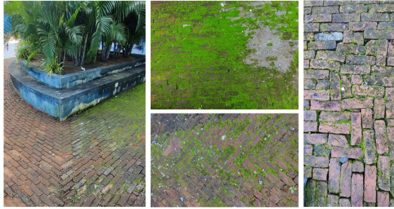
Fig 2. Clockwise from Left - Experimental Sample Vs Controlled Sample, Integration of moss and vegetation in crevices of brick pavers, Cracked and loosely packed brick pavers enabling more vegetal growth (Source: Aswin Senthil 2022)
