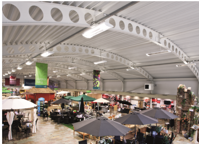
Figure 1 Curved castellated beam in public building (IMAGE SOURCE: http://www.steelconstruction.info )
