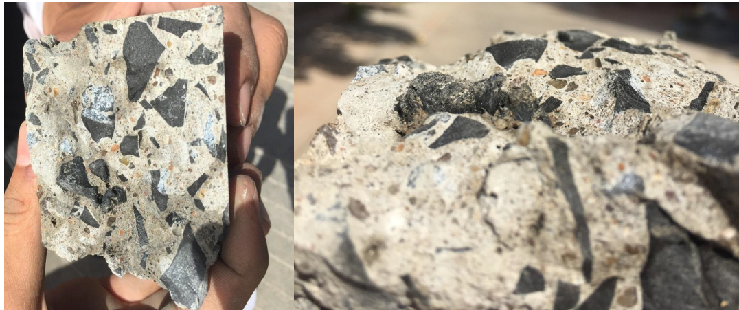
(a) Natural aggregate chipped out
